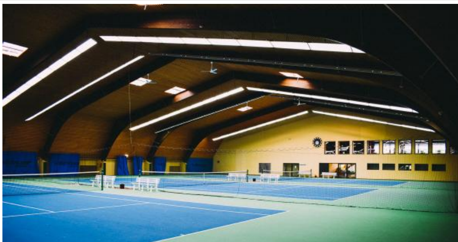
The Racket Arena operates 8 tennis courts and 4 badminton spaces with automated building technology. © Racket Arena Rhein-Erft GmbH & Co KG
